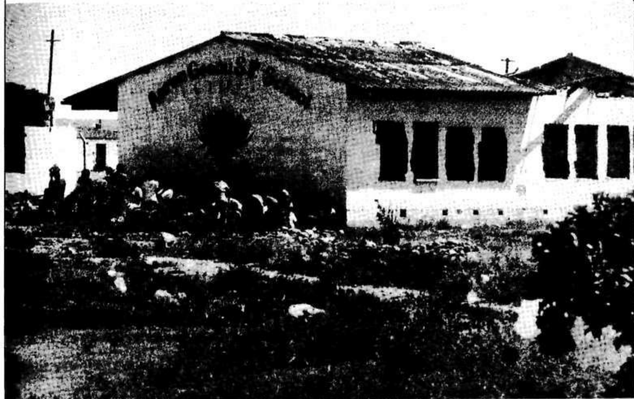
Students have returned to school but the DET has not repaired the classrooms
