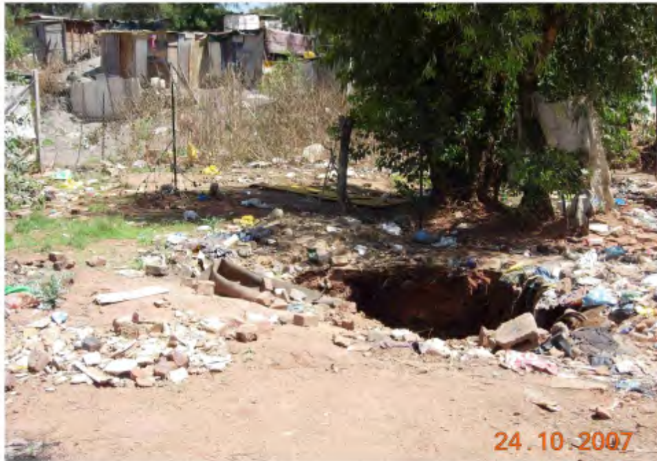
Plate 1. Opening to the mine shaft which measures 4m x 2m.
