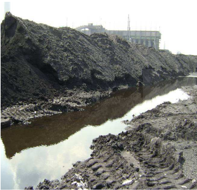
T1-05: Water ponding at the coal storage area
