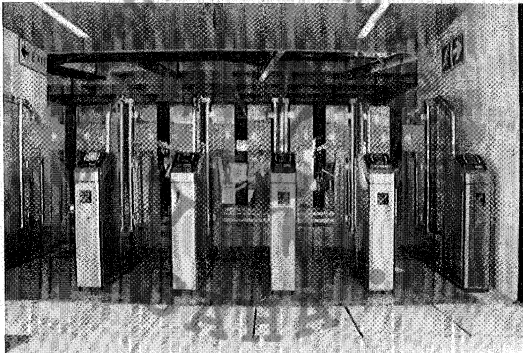
Figure 4 - Access gates at stations
